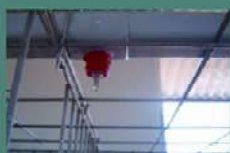
Nipple & PVC Pipe with Saddle
